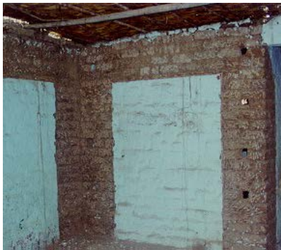
Fig. 3. Sequence of reinforcement on an existing house: Remove the existing cover and perforate the wall (left), connector wire and wire mesh installation (middle), and final cover (right).
