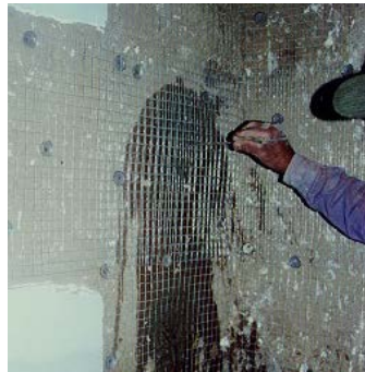
Fig. 3. Sequence of reinforcement on an existing house: Remove the existing cover and perforate the wall (left), connector wire and wire mesh installation (middle), and final cover (right).
